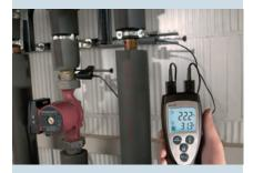
**Solution:** Measurement of the difference between flow and return temperature in preparation for hydraulic balancing.
