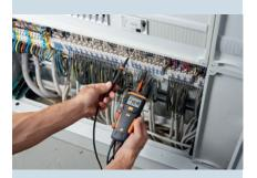
**Solution:** Measure the current and voltage in the control cabinet, on heat pump systems, compressors and air conditioning systems.
