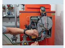
**Solution:** Check the ionization current using a certified multimeter.
