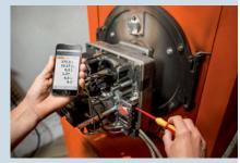
**Solution:** Measure flue gas losses and emission values (CO, CO<sub>2</sub>) and, if necessary, determine the need for maintenance work.
