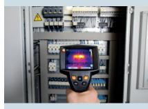
**Solution:** Electrical maintenance with a thermal imager.
